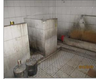
Photo of non-conformity 7.22 Male toilet not equipped with privacy door.JPG
