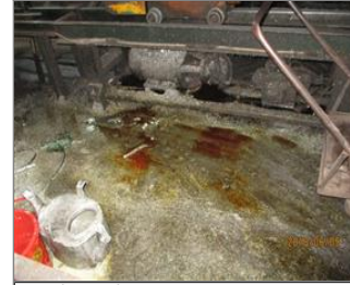
Photo of non-conformity 7.7 Lubricating oil leakage on floor.JPG
