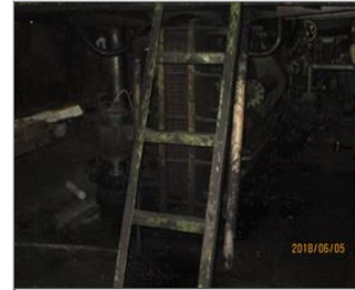
Photo of non-conformity 7.17 Stepladder not equipped with handrail.JPG
